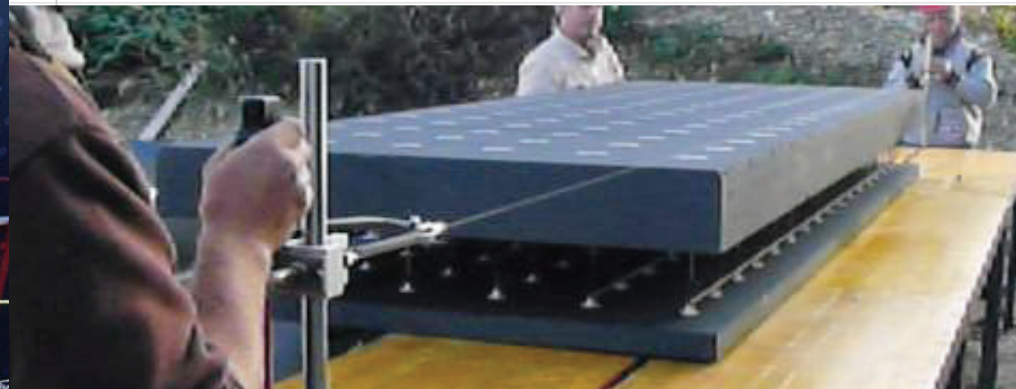
Cutting of formwork element in-situ - same cutting can be done manually by normal wood saw
