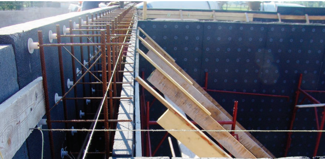
Detail of the rib for floor grid
