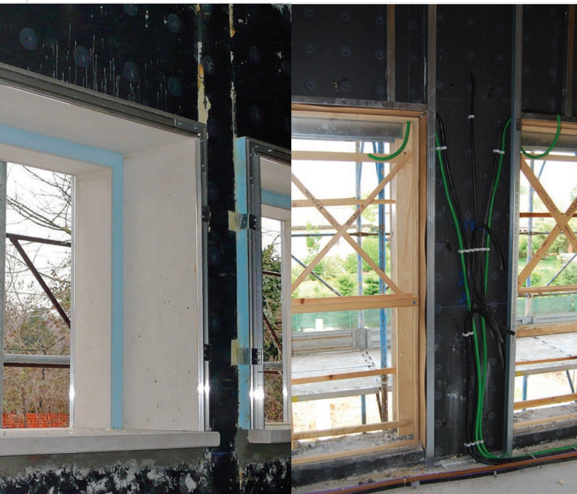
Prefab sub-frame to be mounted before casting
