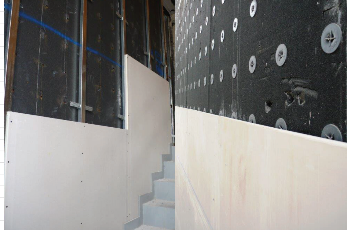
Plasterboard mounted on a structure
