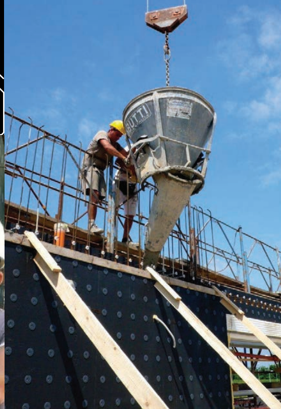
Casting with bucket
