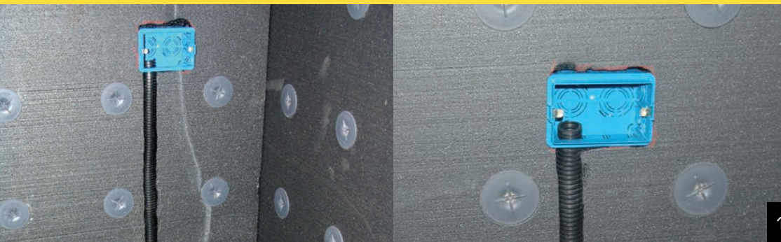
Installations, ducts on the Wall Plastbau® 3 internal panel
