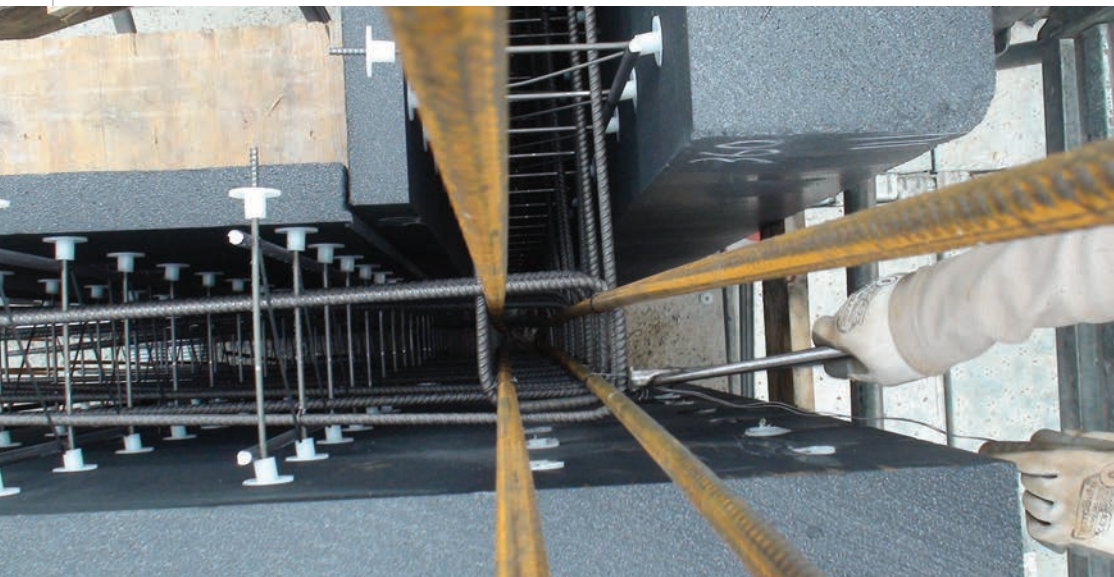
Semi-open corner node / reinforcement
