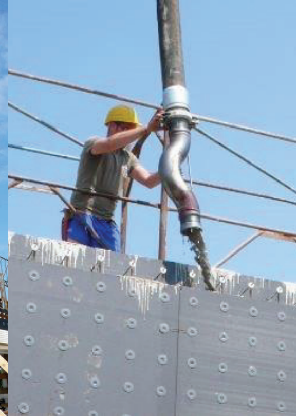
Casting with pump
