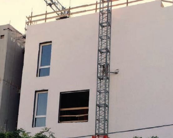
External insulation shaving finish
