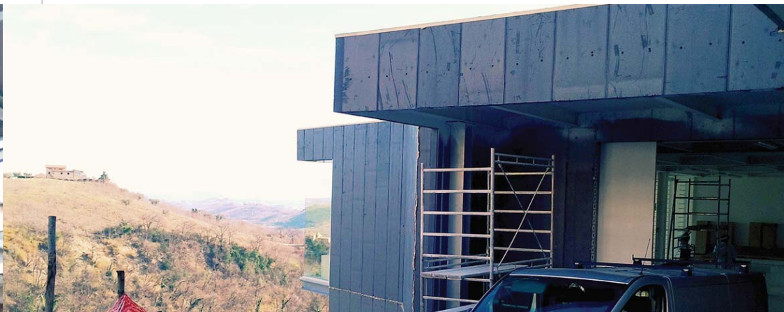
Posa pannelli in divisori
