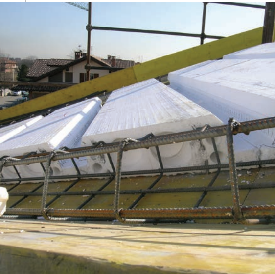
Roofing of a new building
