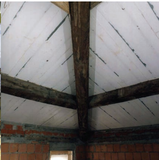
Roofing of a historic building
