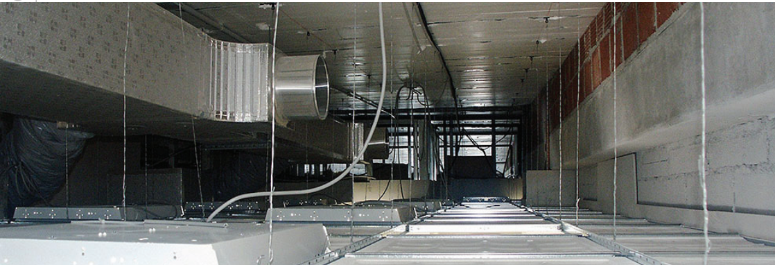
Lowered and dropped false ceiling
