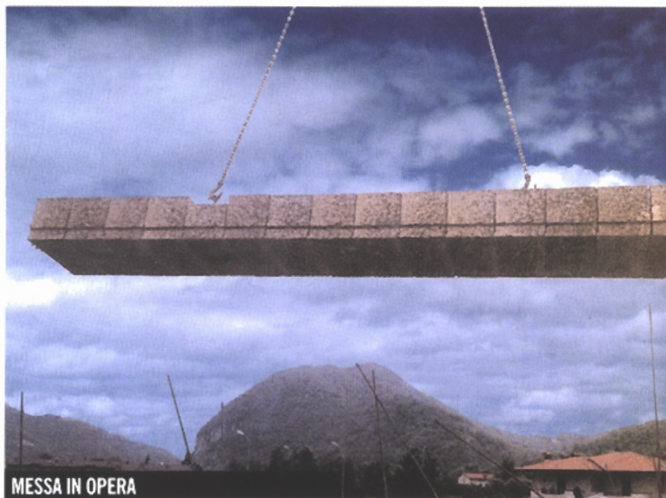
MESSA IN OPERA
